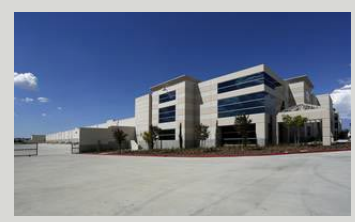
6. SRG Perris Logistics Ctr - Bldg 2
