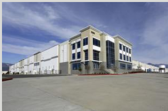
4. Redlands Logistics Center
